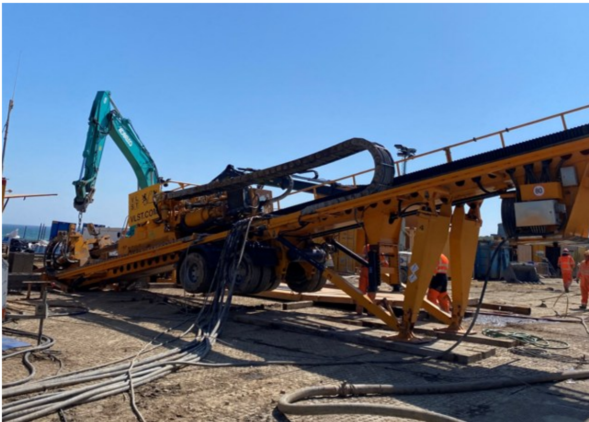
Figure 4.2425: Example of HDD Rig
