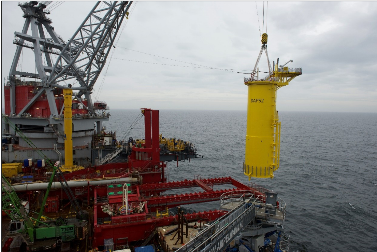
Figure 4.2223: Offshore TP installation (Photo courtesy of Dogger Bank Windfarm)
