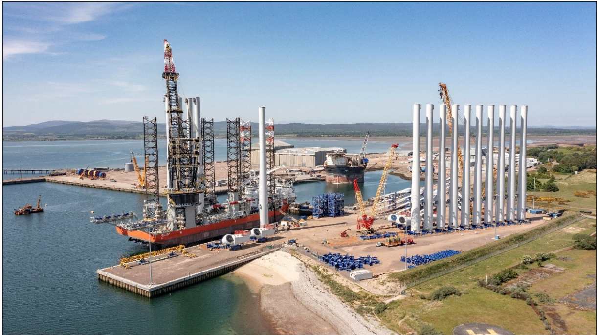
Figure 4.2829: Construction port at Nigg (Photo courtesy of Seagreen OWF)
