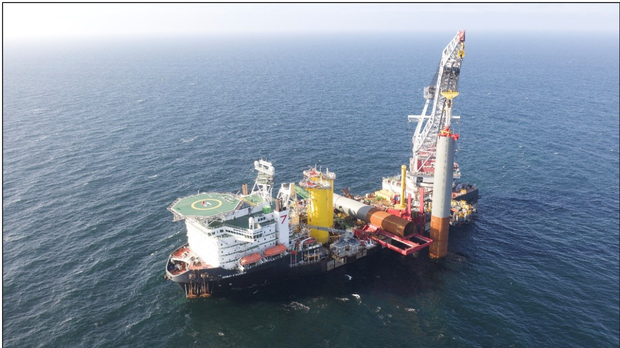
Figure 4.2122: Monopile Installation (Photo courtesy of Dogger Bank Windfarm)
