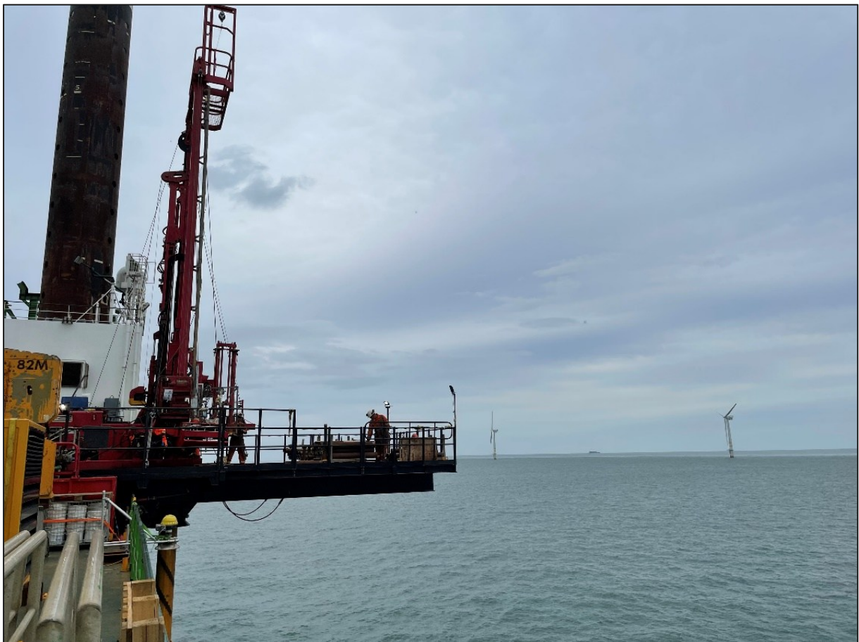
Figure 4.4819: Borehole drilling rig at Arklow Bank
