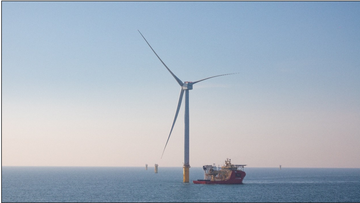
Figure 4.2324: Installed offshore WTG with Monopile and TP installations in background (Photo courtesy of Dogger Bank Windfarm)
