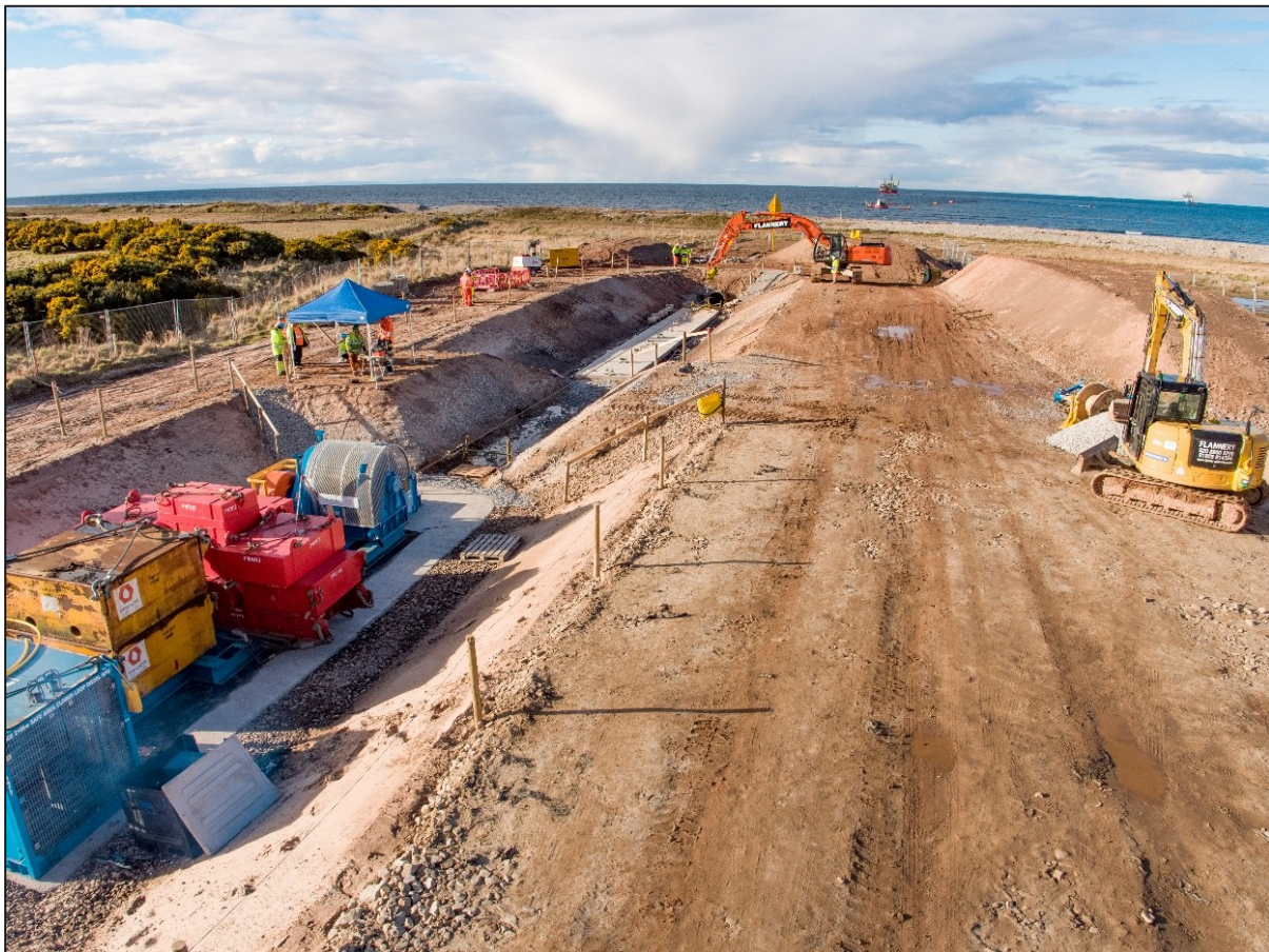
Figure 4.2627: Offshore cable pull operation (Photo courtesy of Beatrice OWF)
